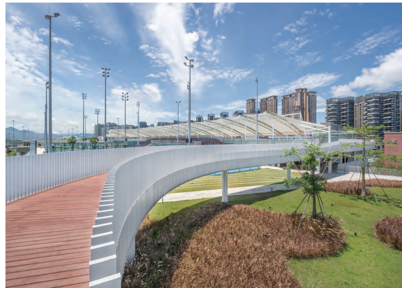
人行天桥 Elevated pedestrian path
